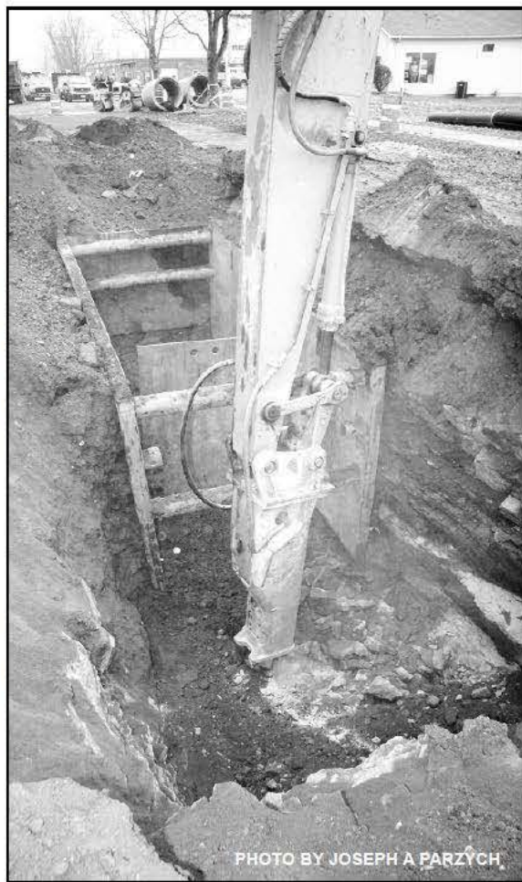
Allied breaker jackhammering on Avenue A after the ledge is softened up by drilling 4 inch holes 18 feet deep, two feet apart. Watch out for that sewer main!
