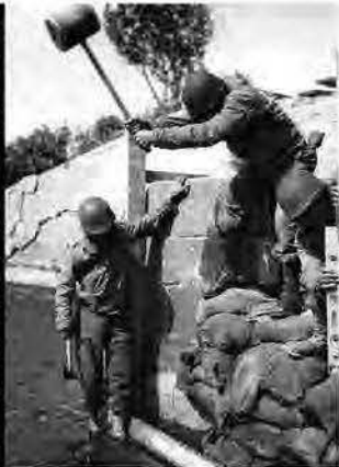
300th Combat Engineer Battalion repairing the under piling of a bridge destroyed by enemy fire along the Carentan - Cherbourg Road in France - June 30, 1944.
