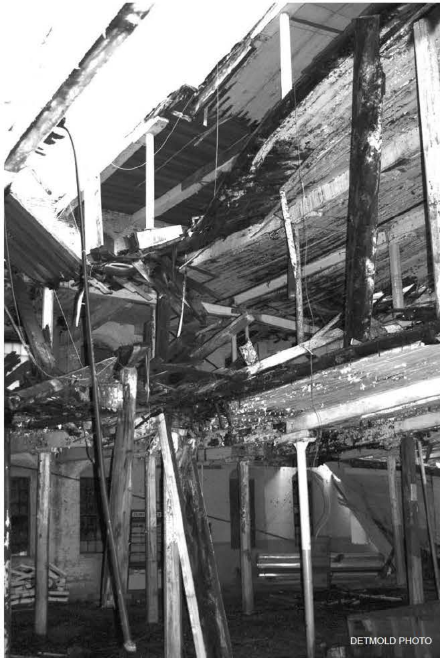
A developer's dream or a neighborhood nightmare? This shot of the collapsed roof and five demolished floors - leading to a dangerous drop to the basement - was taken through the unsecured rear door of Railroad Salvage earlier this week.
