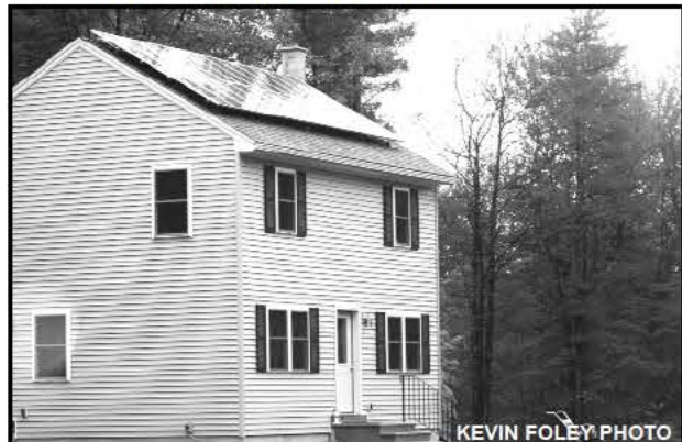
Solar panels top the roof of this Old Stage Road home.
