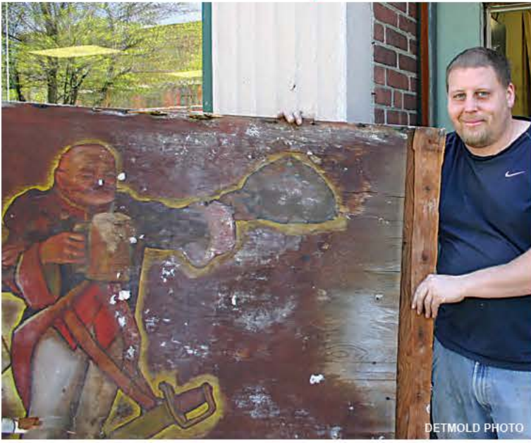
Zak Kelly, of Estes Builders in Buckland , holds a painted panel found behind a wall of the storefront being renovated for Nina's Nook on the Avenue, next to Equi's . Anyone with information about the painting's origins, get in touch.
