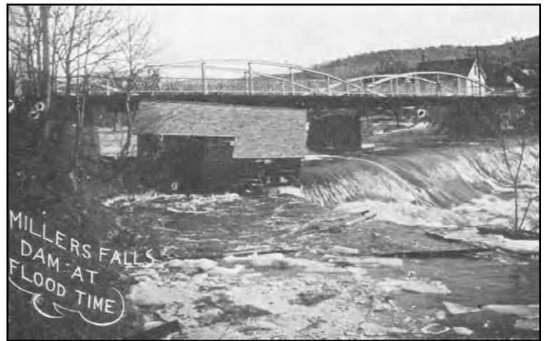
This represents a later view, with part of the mill building no longer there
