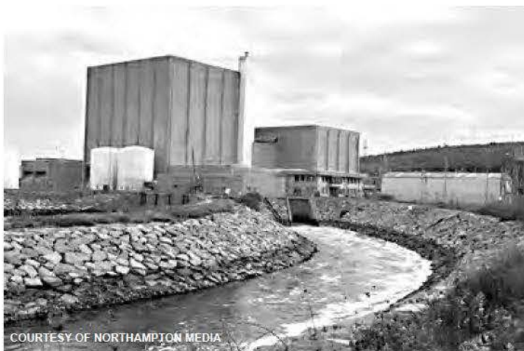
The Pilgrim nuclear power plant in Plymouth, MA
