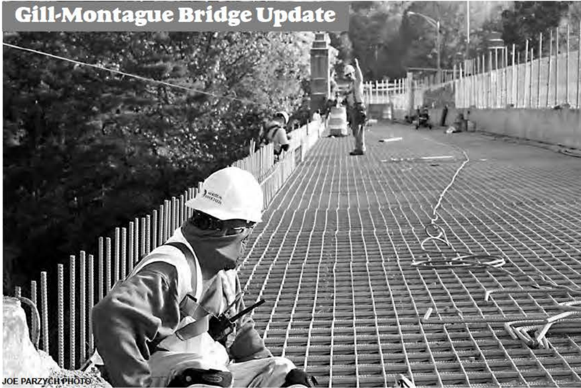
Workers align galvanized grids in preparation for a concrete pour on the Gill-Montague Bridge
