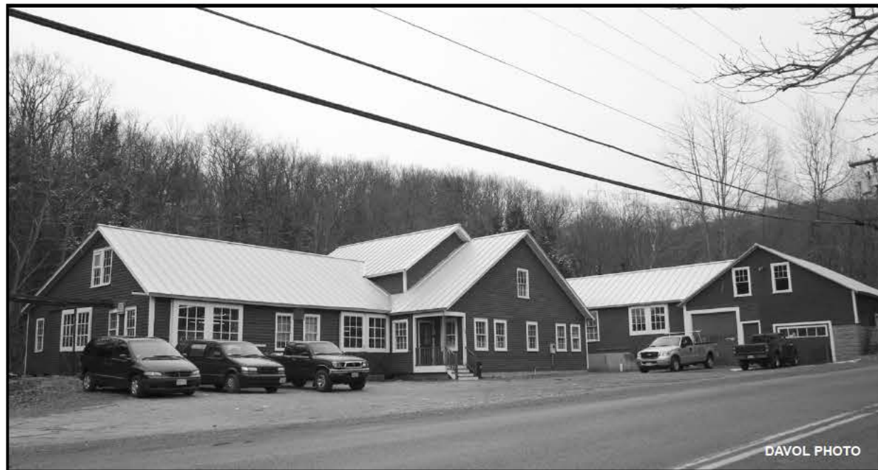
The former Billings-Brown boxshop on North Leverett Road is now the home of Architectural Components, a reproduction and custom window manufacturer. Much of the land beyond was preserved by Woody Brown.
