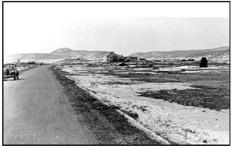
The village of Greenwich, MA after demolition - one of the four drowned towns to be discussed during the Creation of Quabbin Reservoir program by J. R. Greene at Erving Public Library on Tuesday, March 21st at 7 p.m.
