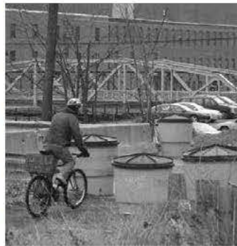
A cyclist enjoys the obstacle course at one end of the Power Street bridge
