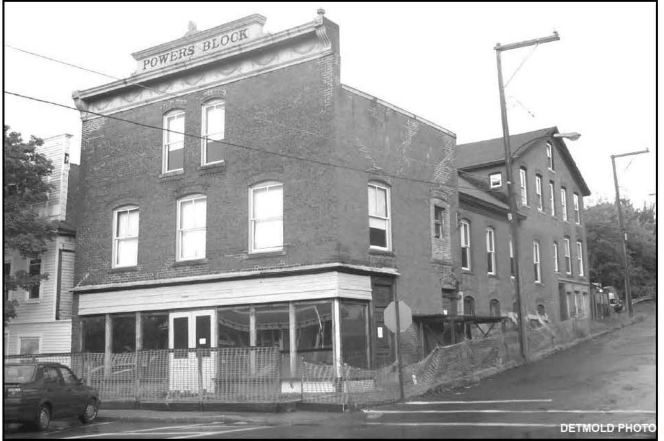
The Powers Block building in Millers Falls
