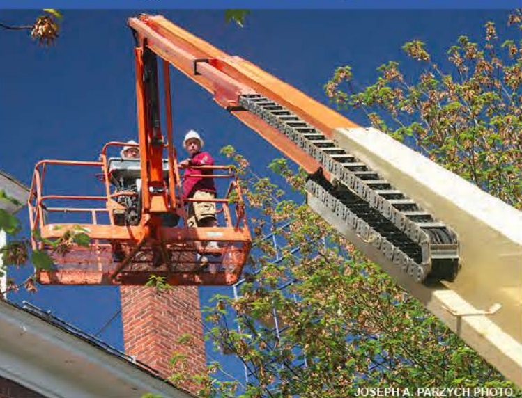
Employees of James Gang Construction remove rooftop sections of a chimney from a Power Town Apartment building on 4th Street
