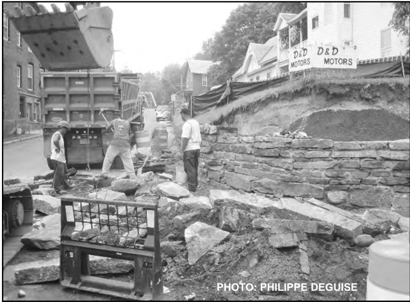
Construction work has begun on the long awaited Millers Falls Streetscape. Here, workers reconfigure the stone retaining wall in front of D&D Motors, widening the intersection at the corner of Main and Bridge streets.
