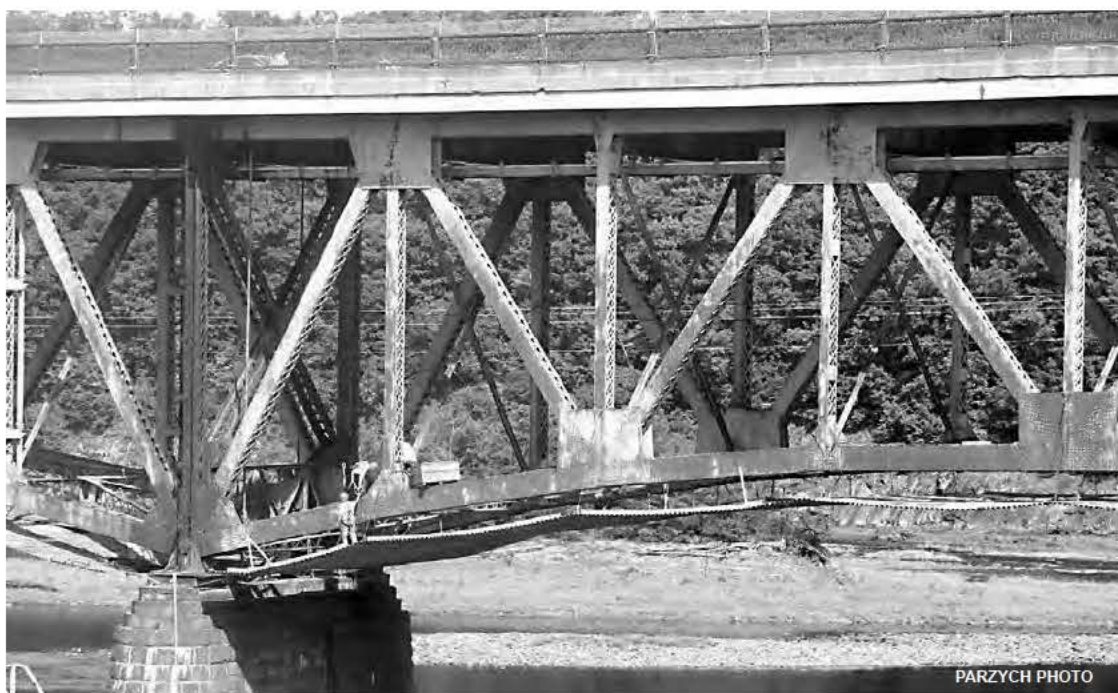
Both the concrete beams and steel girders on the Gill-Montague Bridge are badly deteriorated. Workmen are shown here constructing the work platform under the bridge.
