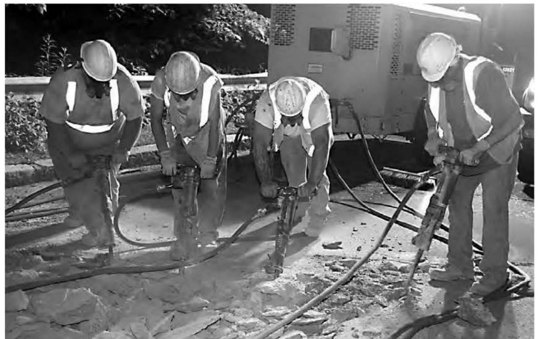
SPS workers demolish deteriorated concrete under the floodlights.
