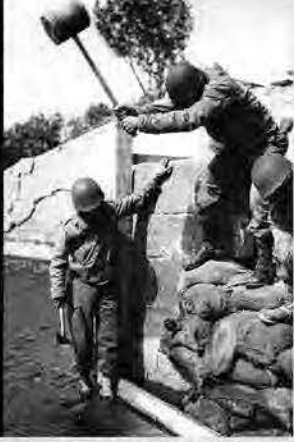
300th Combat Engineer Battalion repairing the under piling of a bridge destroyed by enemy fire along the Carentan - Cherbourg Road in France - June 30, 1944.
