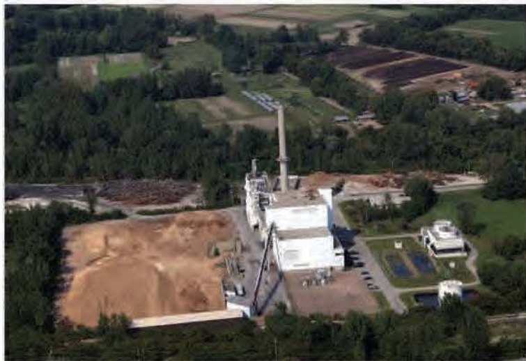
McNeil Station, Burlington, VT (50 MW biomass plant)
