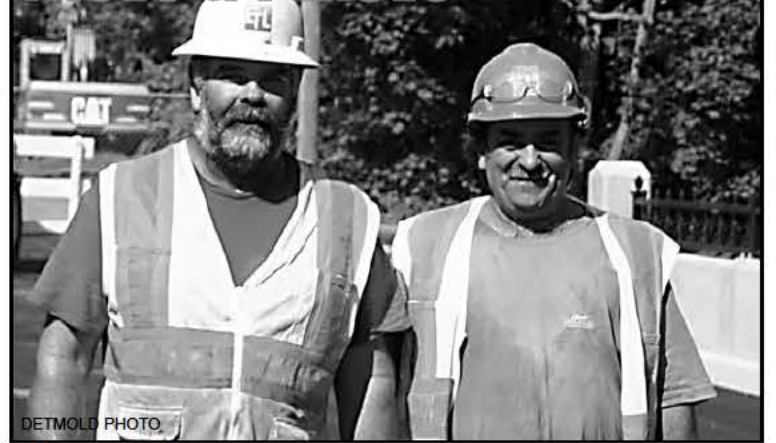
Rich Bradley, (left) ET&L's super on the Prospect Street Bridge replacement in Turners Falls, stands on the completed span with expert laborer Joe Alves. The bridge will reopen Friday, after being closed for more than ten years.
