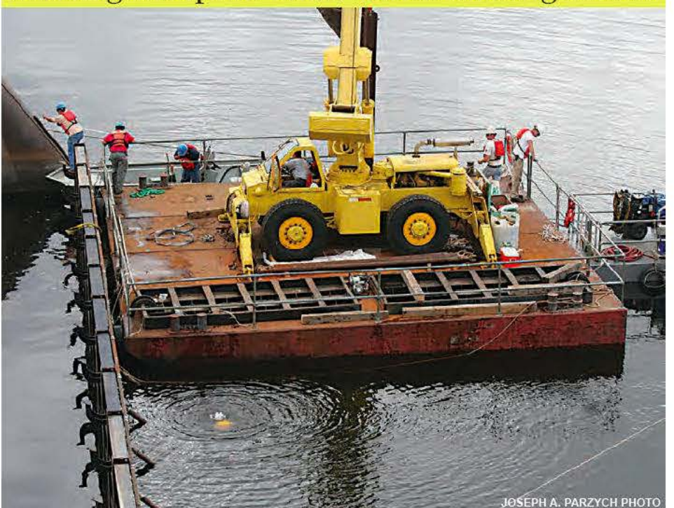
A diver surfaces at the coffer dam as FirstLight repairs leaks in the Gill-Montague dam.
