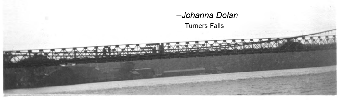
[This poem was written by Francis Dolan's mother, Johanna, after the bridge was dismantled in 1942. The Old Red Bridge, built in 1878, was a smaller version of the Brooklyn Bridge and built by the same engineer - both were suspensions. The abutments stood some 400 feet above the dam.]
