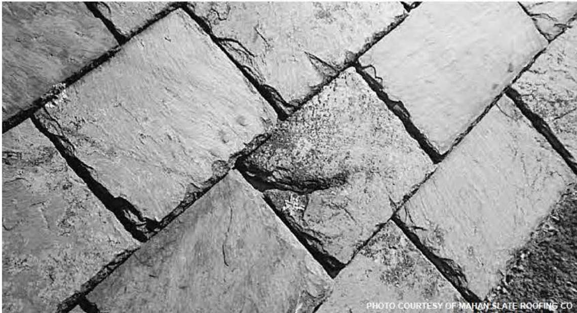
The slate roof at Leverett Elementary is in need of preventative maintenance, at least, to replace damaged tiles.
