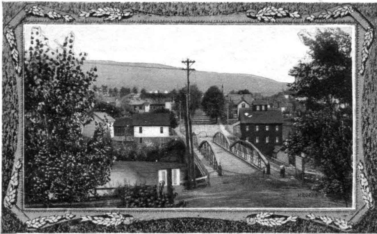
BRIDGE ACROSS THE MILLER RIVER, MILLERS FALLS, MASS.
