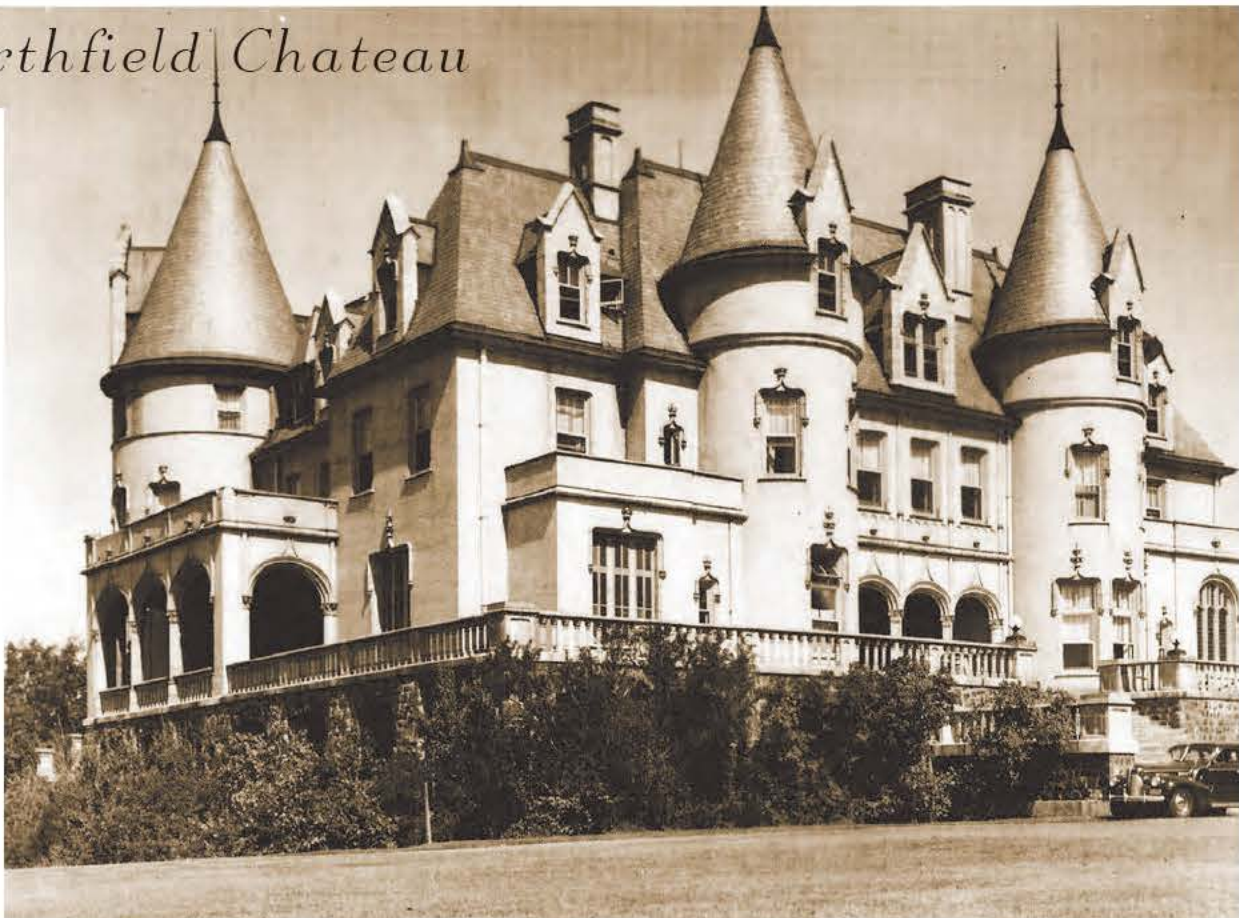
The Schell Chateau, in Northfield, circa 1941, photograph courtesy of the Northfield Historical Society
