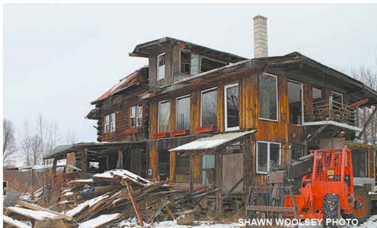
The Franklin Country Land Trust will clean up the Beauchesne property
