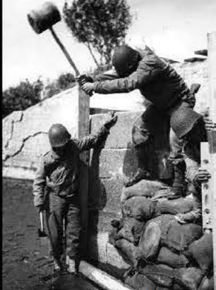
300th Combat Engineer Battalion repairing the under piling of a bridge destroyed by enemy fire along the Carentan - Cberbourg Road in France - June 30, 1944.
