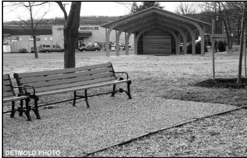
The renovation at Peskeomskut Park has created several problem areas in terms of accessibility including the pea stone walkways and wood chipped play area.
