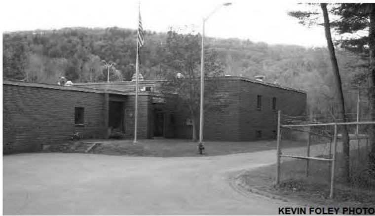
The Erving Wastewater Treatment Plant
