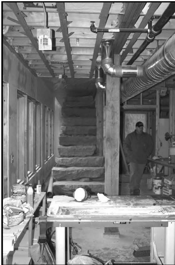
Dairy cows climbed these stone steps to the upper level of the barn for more than a century. The modern facility will be heated geothermally -- with 50-degree water piped from beneath a nearby hillside, year round -- to aid in summer cooling. In winter, the 50-degree water will be used for heat, brought to room temperature with the help of a heat exchanger.
