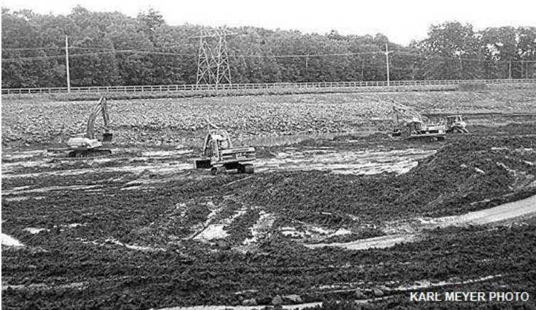
The Power Canal under maintenance; September 2009
