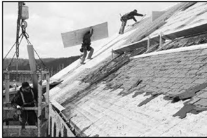
Foreman Michael Campbell, installing metal drip edge, works from the basket as Andy Stevens (left) and Bryan Grunwald (right) place plywood sheathing.
