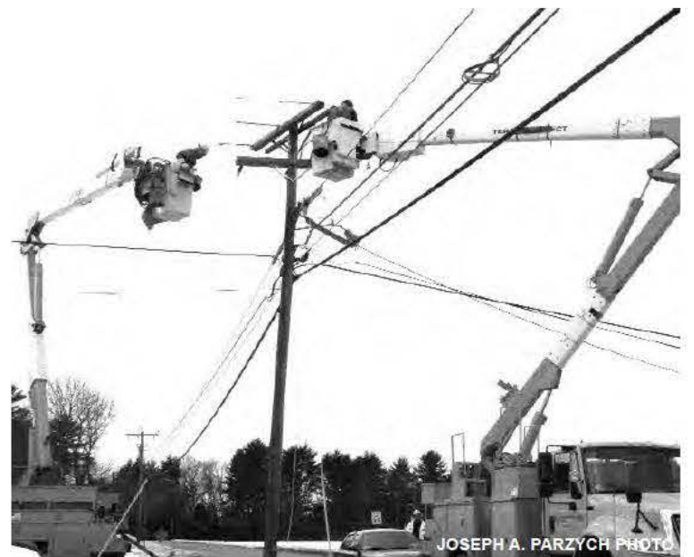
Western Mass Electric Company connected a secondary feed to Riverside in Gill on Wednesday at the intersection of Main Rd and W. Gill Road to avoid Riverside's loss of power every time someone wipes out a pole on Route 2, in Factory Hollow, which happens all too often.
