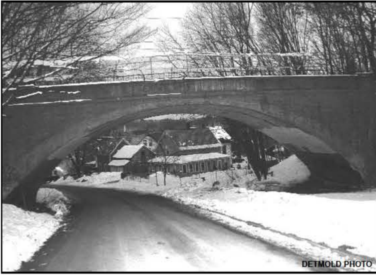
The Prospect Street Bridge
