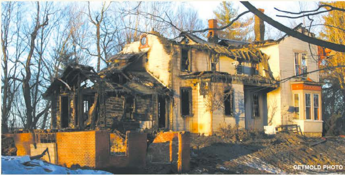
The Dobias - Watroba home on Grand Avenue in Millers Falls was a total loss following a Sunday night fire of unknown origin, that started in the attached barn, at rear.
