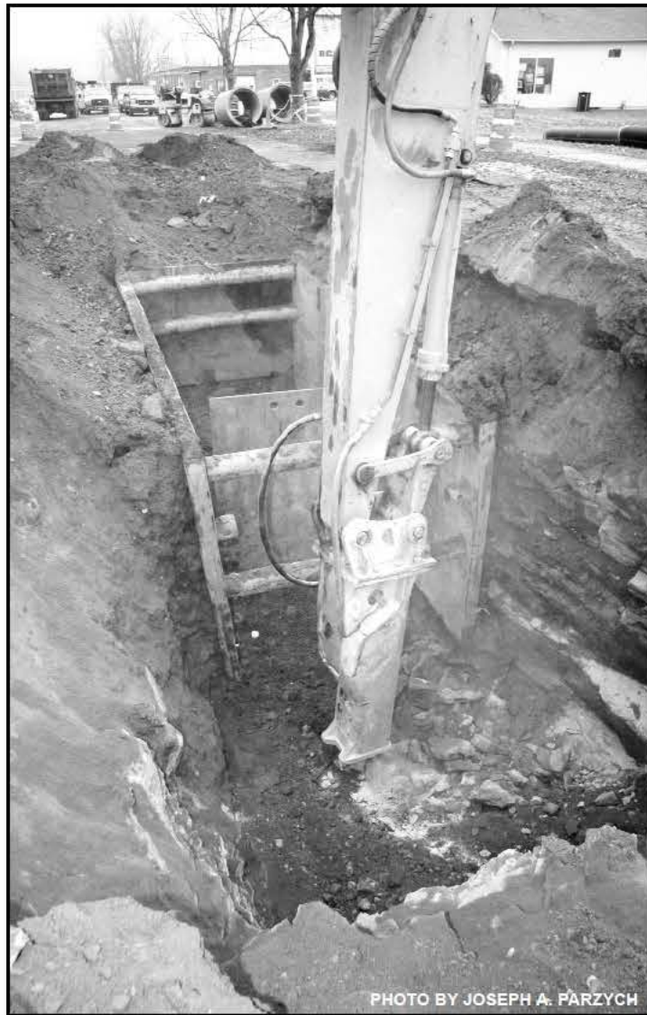
Allied breaker jackhammering ledge after being softened up by drilling 4 inch holes 18 ft deep, two feet apart.
