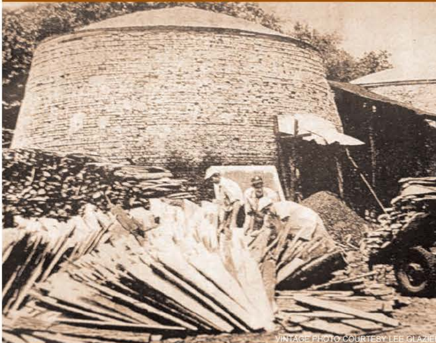
Members of the Howard family begin loading the kiln through the iron door at the bottom, later finishing up at the upper door accessed by an earthen ramp.
