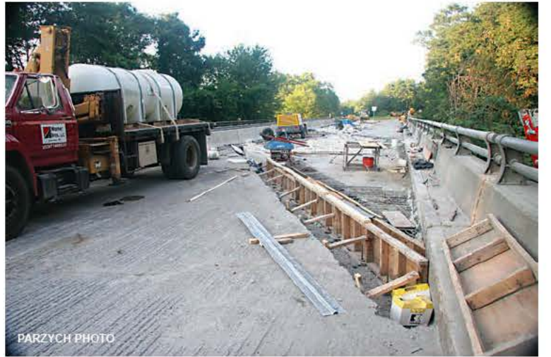
Repair Work in progress over Country Club Road in Greenfield
