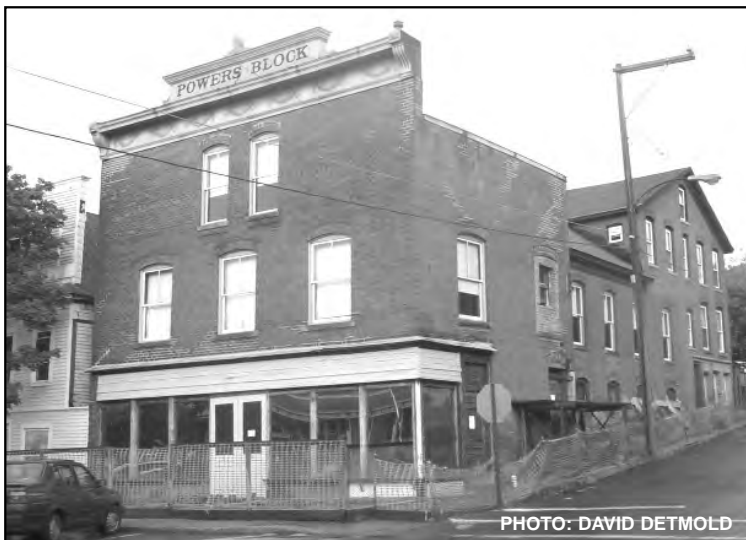
The Powers Block building in Millers Falls
