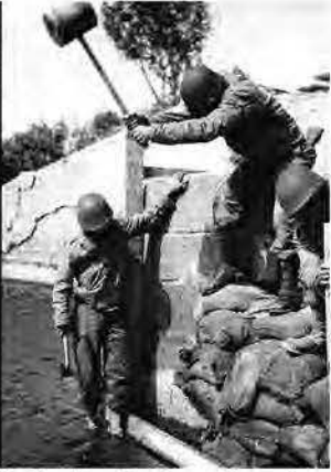
300th Combat Engineer Battalion repairing the under piling of a bridge destroyed by enemy fire along the Carentan - Cherbourg Road in France - June 30, 1944.
