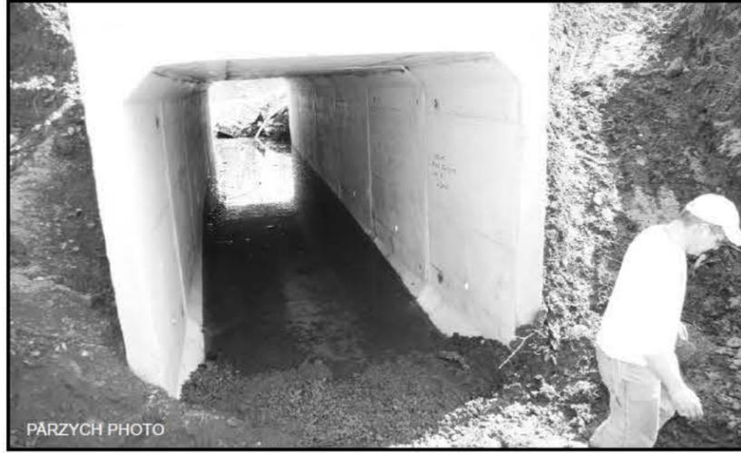
Excavator Joe Fernandes of F&J Construction inspects progress on the box culvert beneath Main Road for the safe passage of wood turtles, a species of special concern in Massachusetts.
