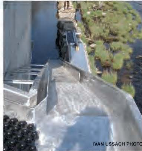
The Orange Eel Pass on the Millers River Black plastic (bottom left) aids the eels’ ascent
