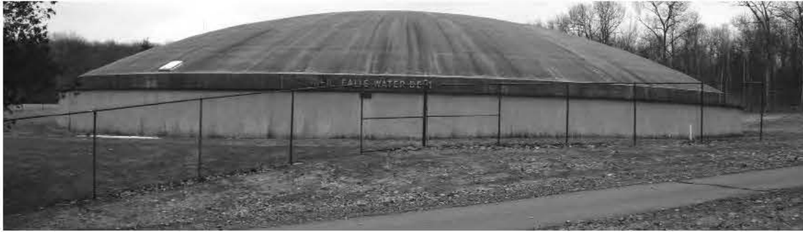
The Turners Falls Water Department's Four Million Gallon Water Tank on Will's Hill
