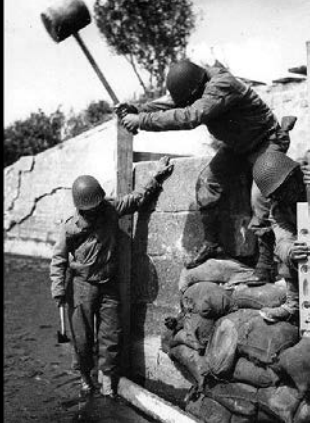
300th Combat Engineer Battalion repairing the under piling of a bridge destroyed by enemy fire along the Carentan - Cherbourg Road in France - June 30, 1944.
