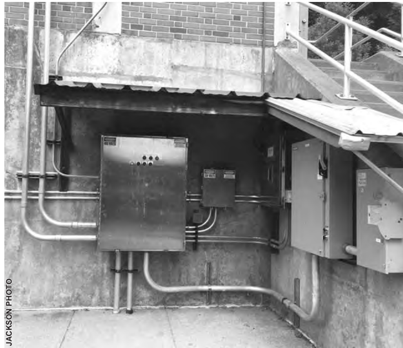
Components in this electrical system were damaged in last Thursday's storm.
