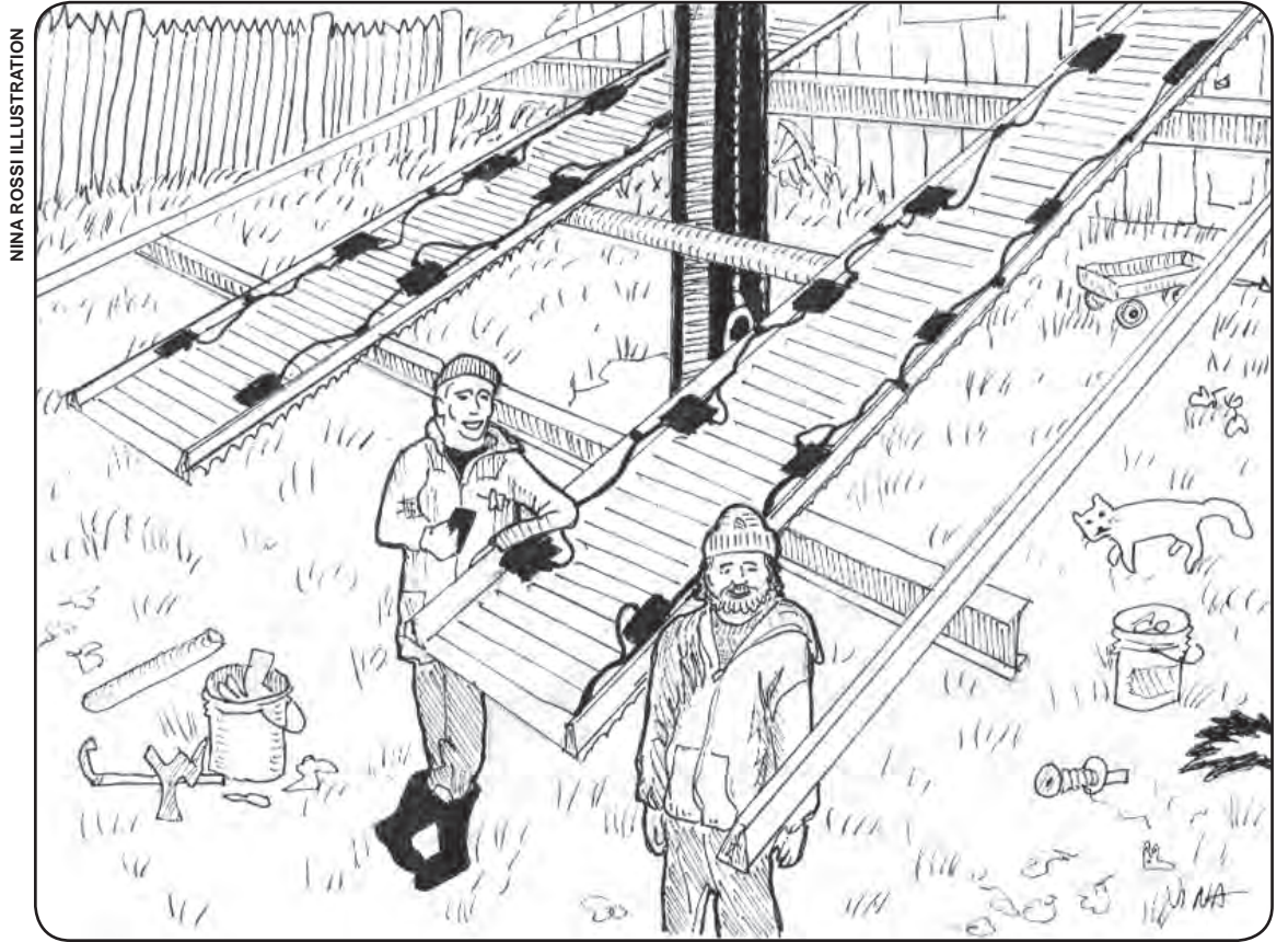
PV Squared solar installers Jeremy Latch and Bob Hiland complete the wiring for a 4.9 KW solar array on Central Street in Turners Falls this Tuesday morning.
