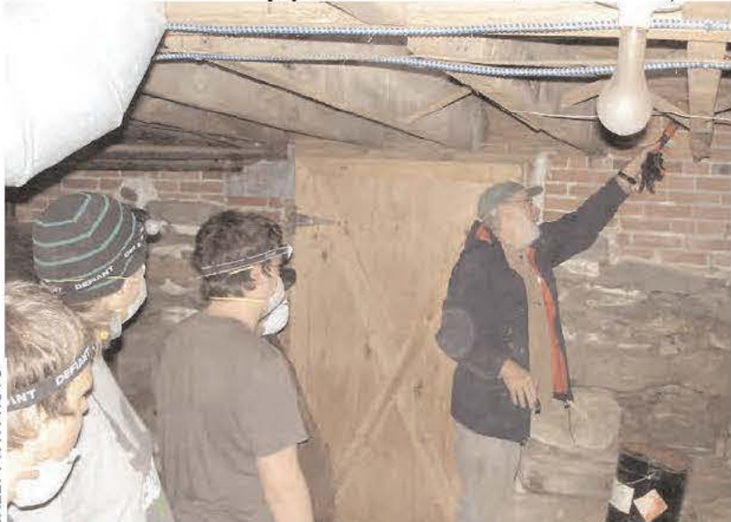
Scott Reed, Co-op Power's lead trainer for the Green Jobs program with the Brick House, shows trainees places to seal air leaks along the sill basement.
