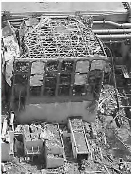
This March 24, 2011 aerial photo shows the damaged Unit 4 of the Fukushima Dai-ichi nuclear power plant, where 1,231 irradiated fuel rods sit in an upper story storage pool.
