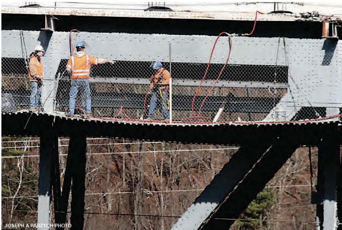
JOSEPH A. PARZYCH PHOTO Work continues on the Gill-Montague Bridge, which will be closed entirely to traffic from 6 p.m. to 2 a.m. on Monday, April 2nd, as SPS New England removes fascia beams and repairs diagonal struts below the deck.
