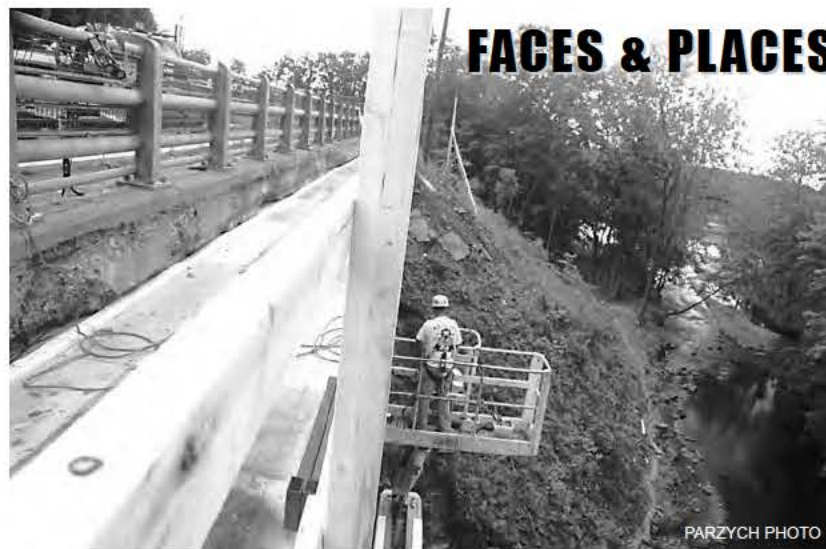
Bill Leb adds more support brackets to the pedestrian walkway of the Gill-Greenfield Bridge from the safety of a man-lift, high over the Falls River. Sidewalk's open. Now, all we need are some pedestrians!
