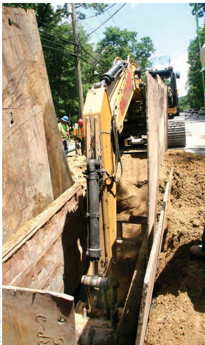
Baltazar Contractors, Inc. use a heavy weight digging box with steel plates, 20 feet long by 8 feet wide, driven down beside the digging box to protect employees who need to get into the trench. On the construction of the original sewer by the Montague Highway Department, there was no shoring of the trench walls.
