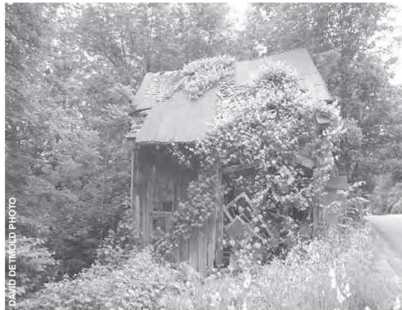
Collapsed barn on Dudleyville Road
