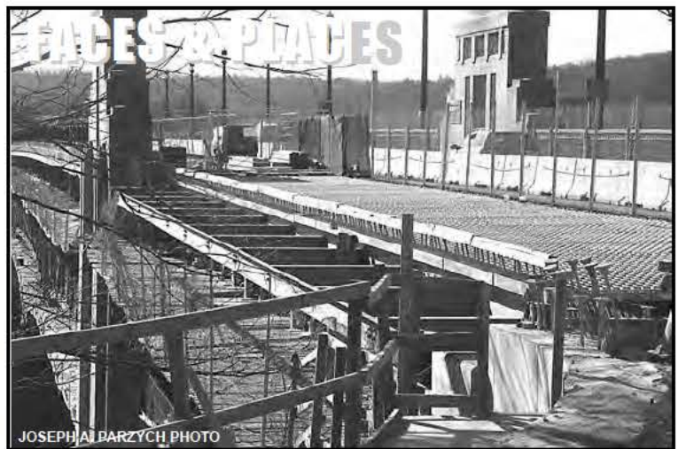
Work on the Gill-Montague bridge has stepped up, with balmy weather appreciated by SPS New England workers replacing rusted beams and putting bridge decking grids in place. In the foreground, cantilevered beams to support the future sidewalk are now in place.
